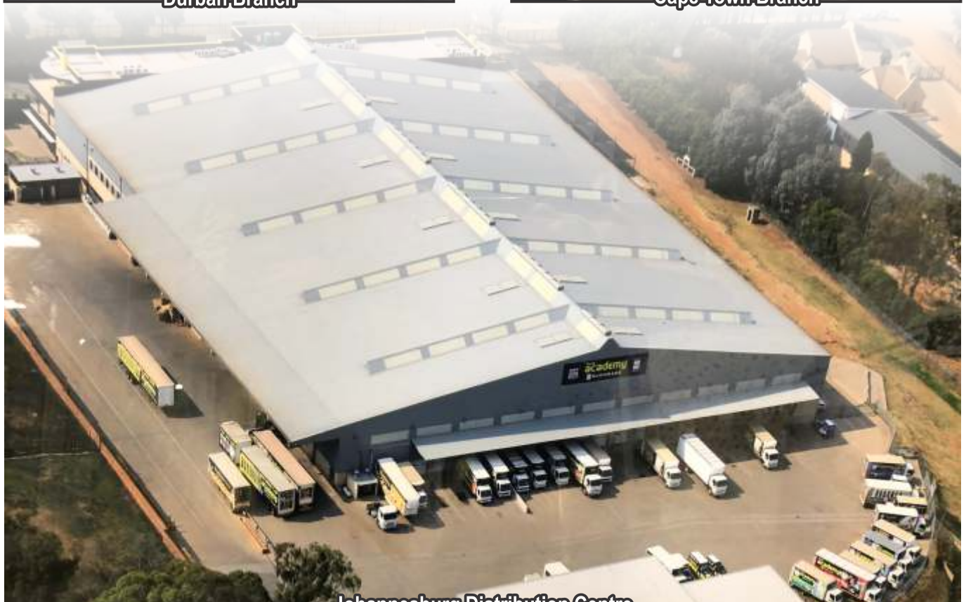
Johannesburg Distribution Centre
